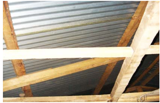
Construction of Kitchen with CGI Sheet is under process
