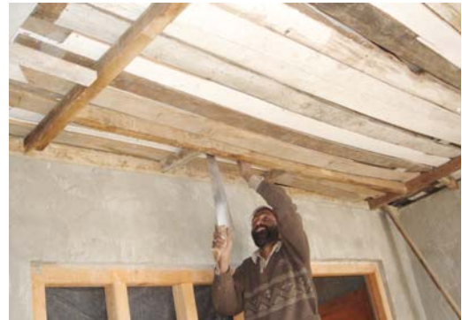
Construction of Kitchen and Washroom at Village Bermong
